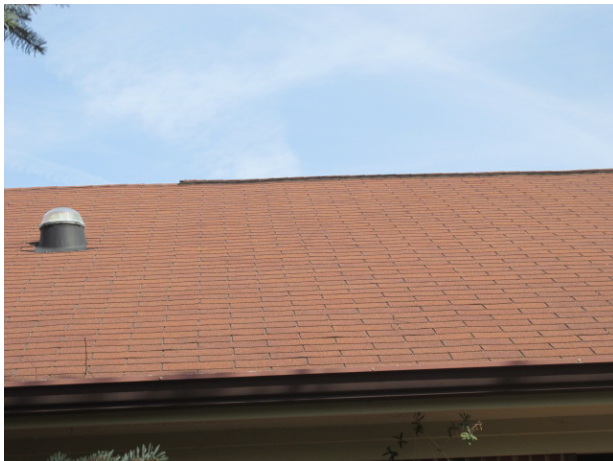
Asphalt shingle roof
