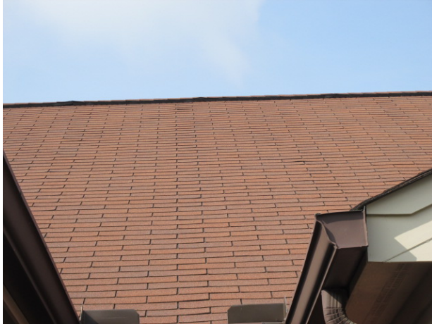
Shingle lift at 2003-2005 Buildings
