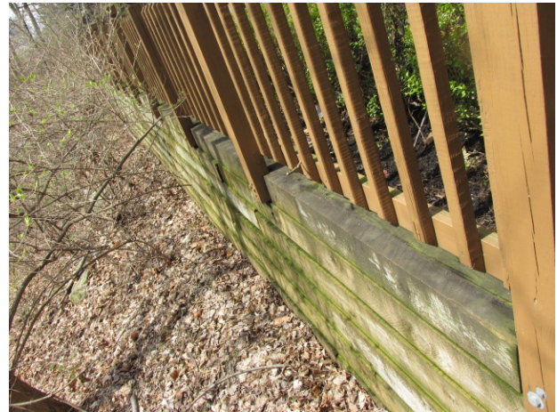
Timber retaining wall
