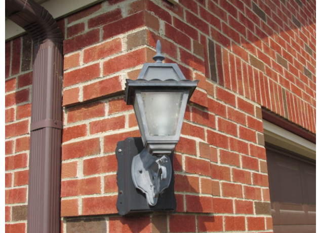
Garage light fixture
