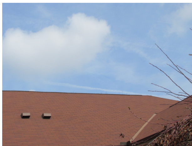
Asphalt shingle roof
