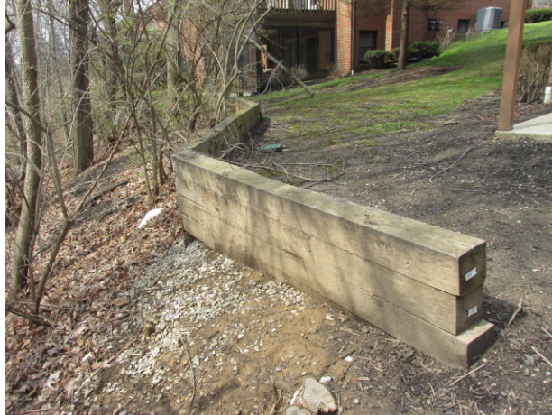
Timber retaining wall
