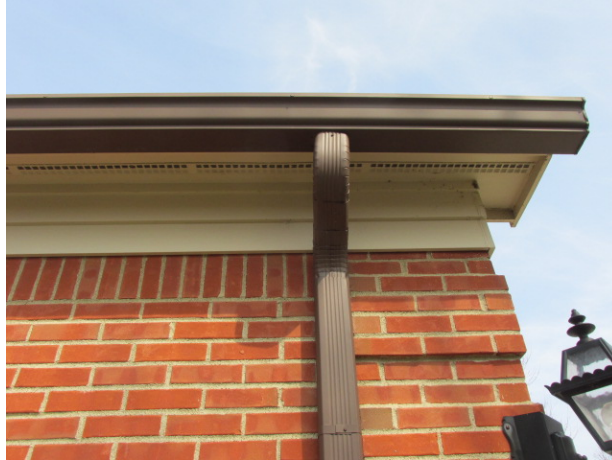
Gutter and downspout configuration
