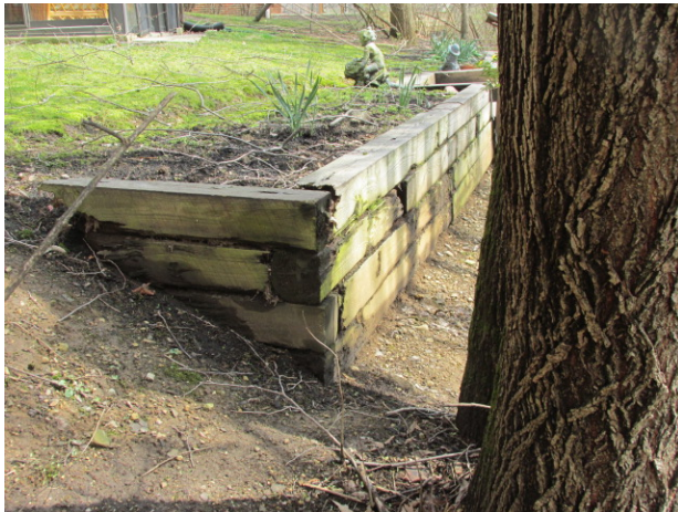
Wood deterioration
