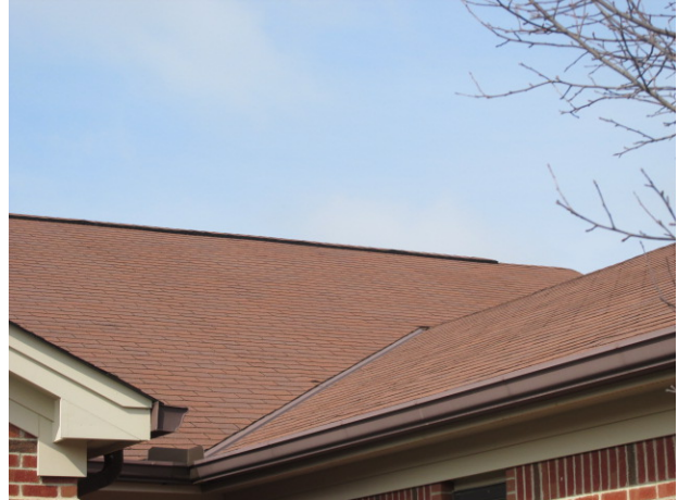
Shingle lift at 2003-2005 Buildings
